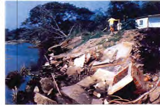
Ablution facilities on the bank of the Mzimba River, Natal, destroyed by river flood
