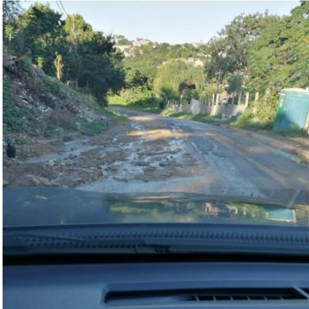
Figure 21. Sewerage leaks in Ward X
