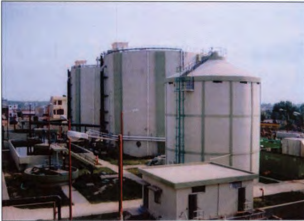
Figure 10 Photo of 1.0 MW power project based on cattle dung at Haebowal Dairy Complex Ludhiana, Punjab (Dhussa, 2004)
