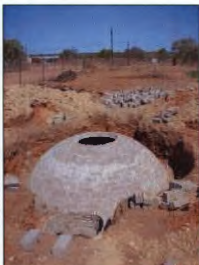
Figure 9 Photo: Rural digester Giyani, Limpopo, 15m 3 feedstock: cow manure (Authors own photo)
