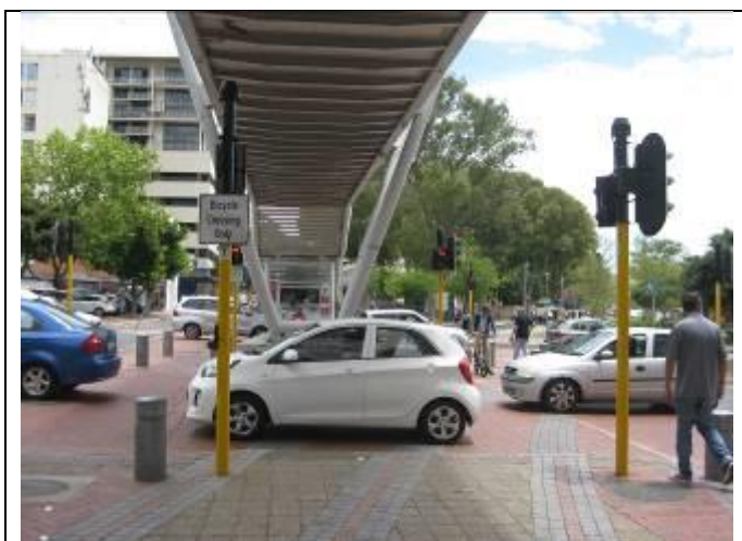
The NMT Crossing facility across Buitengracht Street: The NMT crossing across Buitengracht Street provides traffic signals for pedestrians and cyclists. When the push buttons are pushed, the signals take more than 40s to activate. The time for pedestrians to cross is not enough for users to walk across both carriageway. During the site visit a wheelchair user had to scramble across one carriageway to make it in time. The timing for the pedestrian signal needs to be improved.
