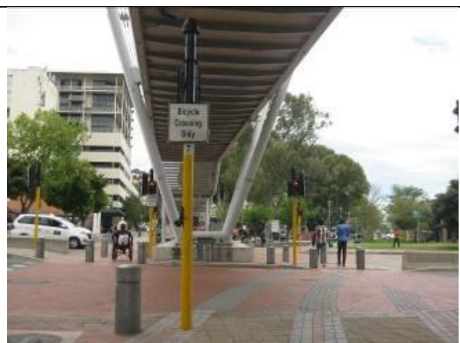
The NMT Crossing facility across Buitengracht Street: From the photo it is observed that a pedestrian bridge is provided for pedestrians. This facility was only used once during a 1.5 hours’ period on site. Most pedestrians crossed at-grade. Vehicles approach the crossing quite fast on Buitengracht Street, which is a Class 2 distributor road. Improvements should be investigated.
