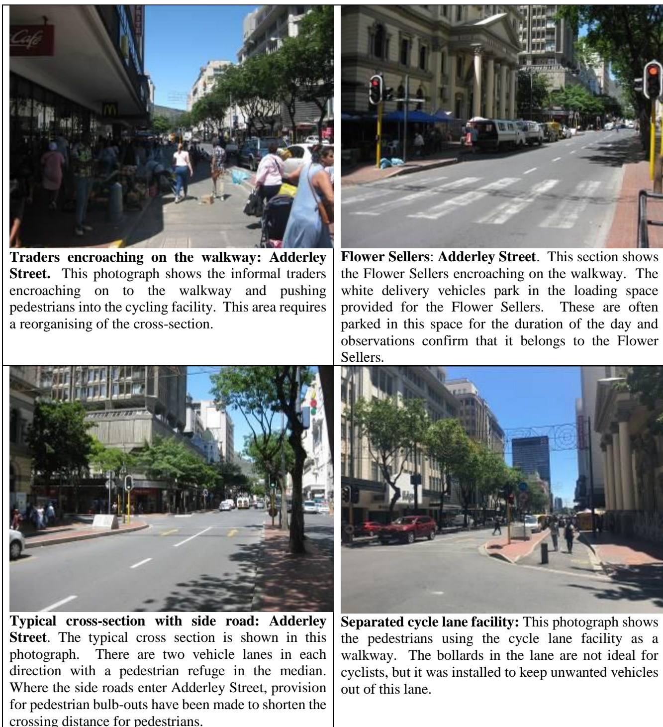
Figure 22: Photos of Adderley Street from the Strand Street Intersection to the Company Gardens. Source: Author’s own.
