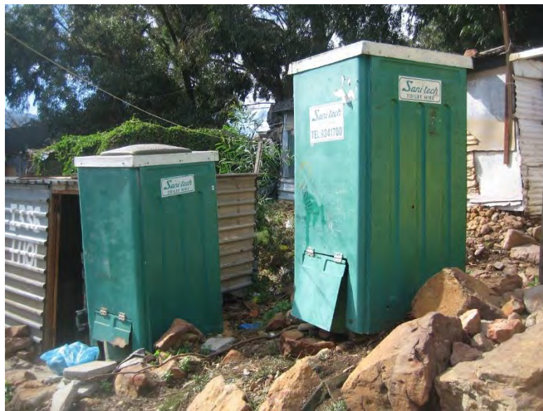
Figure 1. Portable toilets in Imizamo Yethu. The city has provided portable toilets to alleviate the demand for sanitation infrastructure. However, it was reported that they are not used because they do not get emptied on a regular basis
