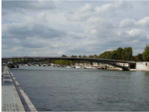
Figure 1.3.: Passerelle Léopold-Sédar-Senghor Bridge in France. (Sun and Yuan, 2008)
