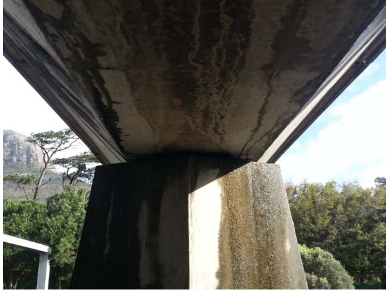
Figure 6.3.: Actual support connection of the Rhodes Memorial Footbridge
