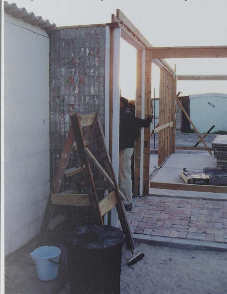
one day to load, transport, + unload the panels - two full days + eight workers to erect all the panels
