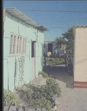
hazel's existing RDP house (single-wall concrete block construction, no ceiling insulation) + 2 shacks
