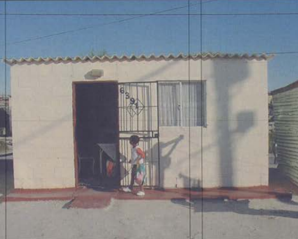
hazel's existing RDP house (single-wall concrete block construction, no ceiling insulation) + 2 shacks
