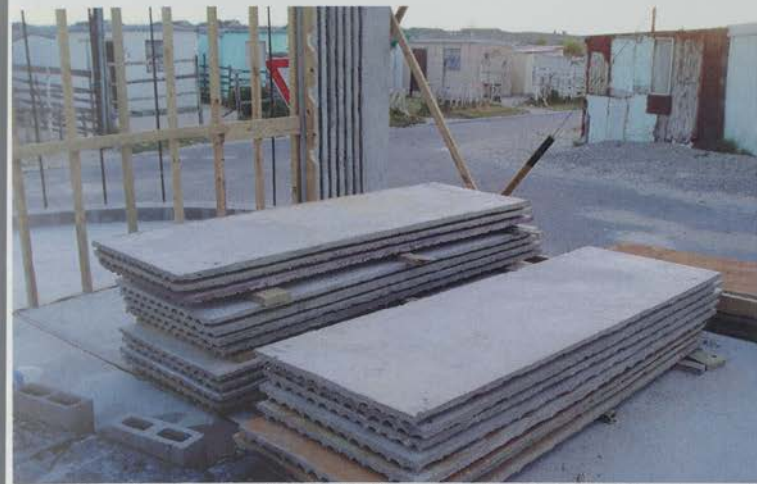
one day to load, transport, + unload the panels - two full days + eight workers to erect all the panels
