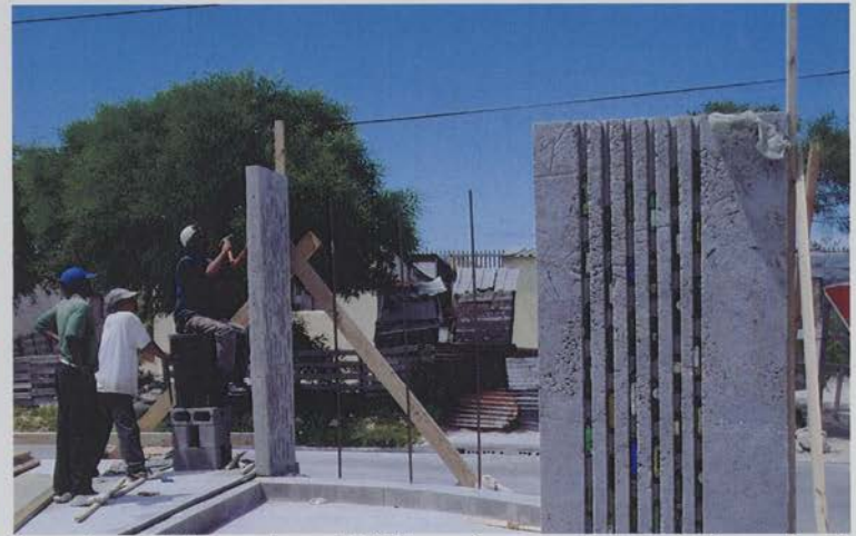
bottle wall, using 'tilt-up' concrete slab method
