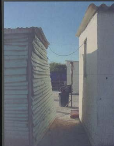
hazel's existing RDP house (single-wall concrete block construction, no ceiling insulation) + 2 shacks
