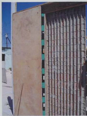
one day to load, transport, + unload the panels - two full days + eight workers to erect all the panels
