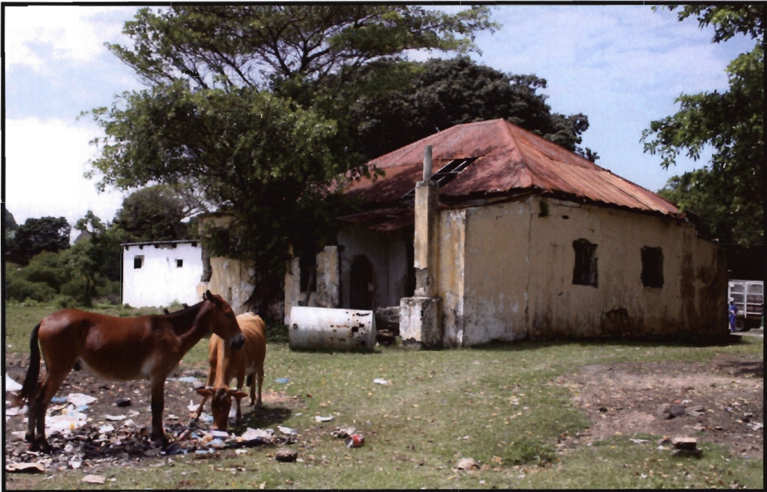
Figure 6.8: During the mid-1980s Transkeian President Kaiser Matanzima took over the running of the Ocean View Hotel and purchased this house, which now lies in ruins as his holiday home. (Author's own collection, 2005)
