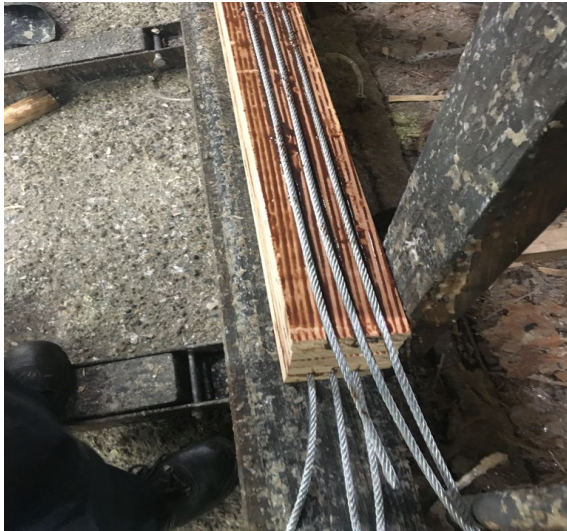
(a) Ø 8mm Cables lying in the grooves
