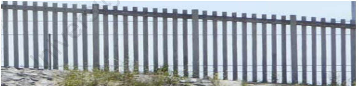
Figure 7.5. Concrete wall separating the townships from the reserve
