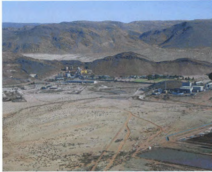
Figure 1.2: A section of the mining area of BMM (Photo courtesy of BMM)
