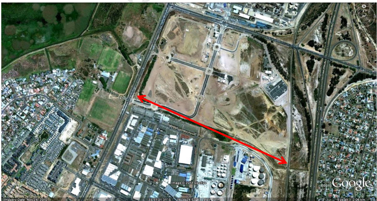
Photograph 3: Aerial view indicating re-aligned stream on southern site boundary (Google, 2011)
