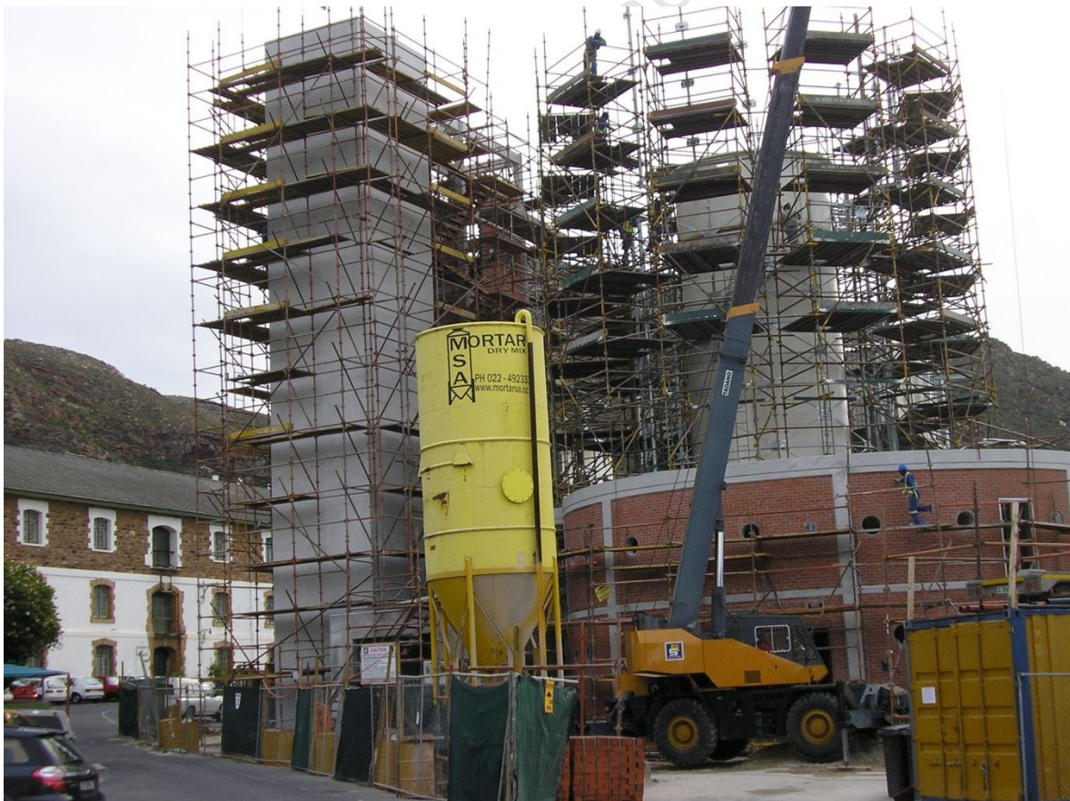
Photograph 7: Simonstown - View of construction in progress (Pillay, 2010)
