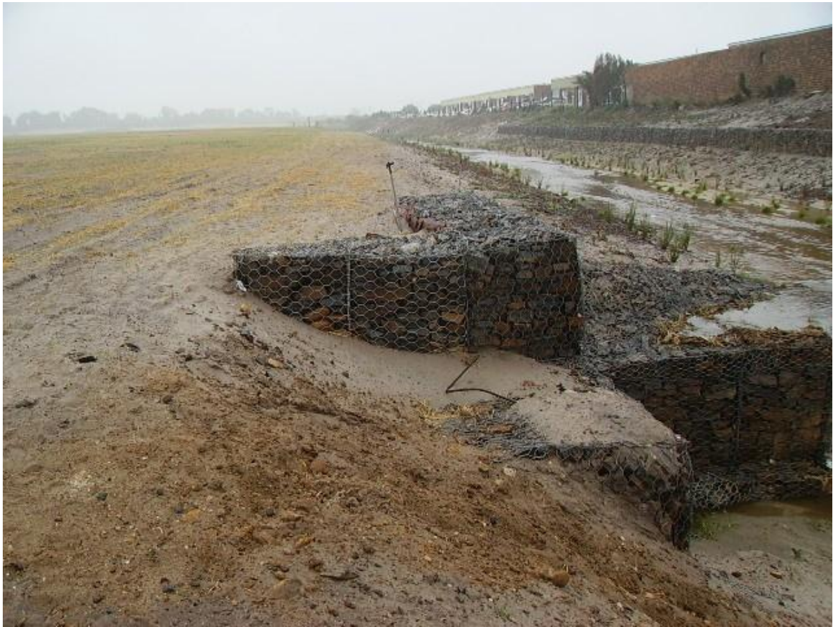
Photograph 4: New water course constructed (Rabie, 2006)
