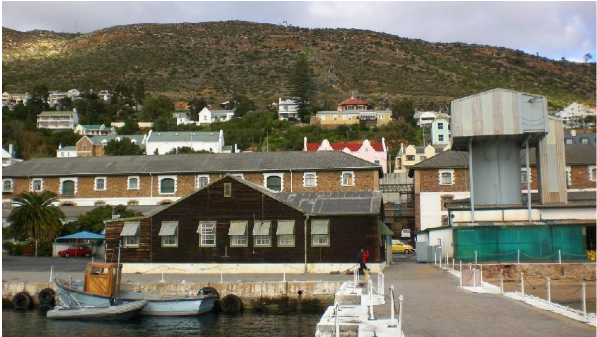
Photograph 6: Simonstown - View of West Yard Diving School before construction (Eitzen, 2008)
