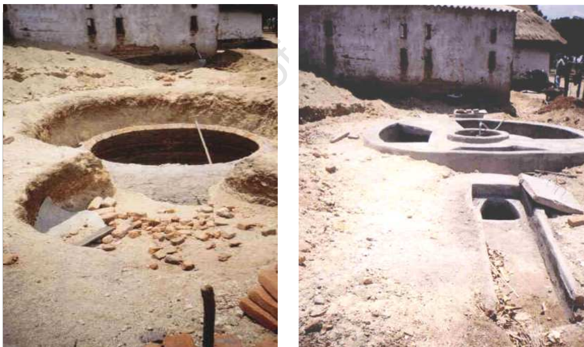
Figure 4.5: Biogas construction plant in Zimbabwe (Mavunganide Kennedy, 2005)
