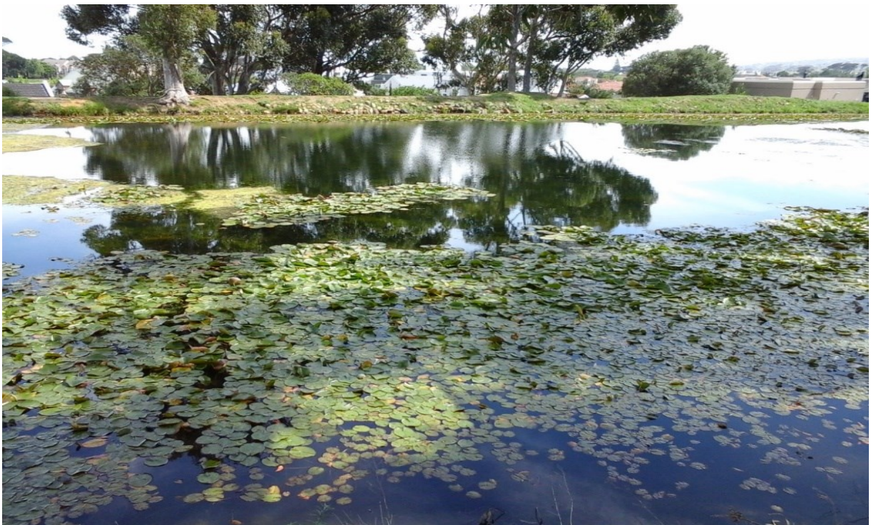
Figure 3-5 A typical retention pond
