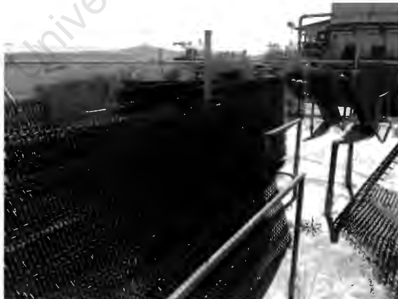
Figure 4.8: Vibrating screens used to sieve materials at the AFRISAM plant at Peninsula Quarry. Wire mesh screens with elongated apertures used to remove flaky particles at the AFRISAM plant
