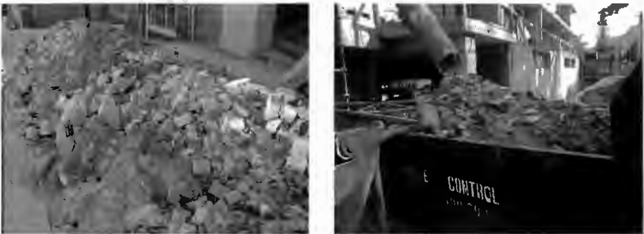
Figure 2.6: Stockpiles of mixed C&D materials in Cape Town
