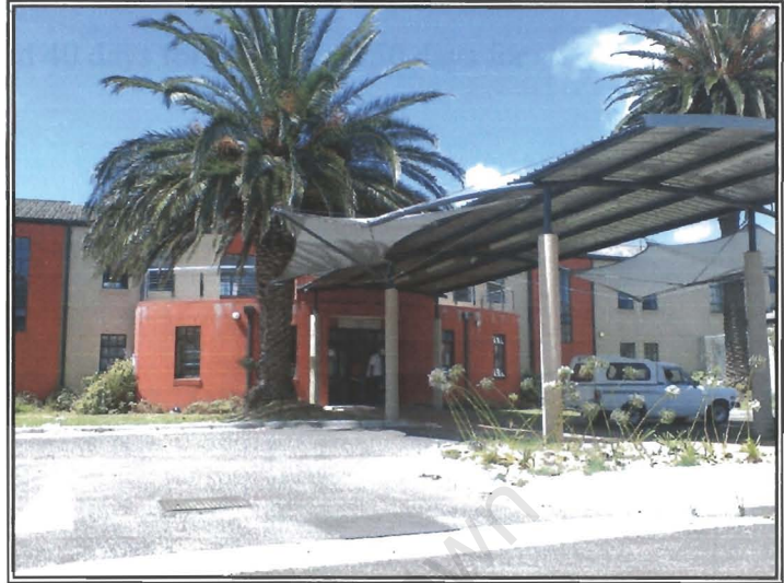
Figure 1: Valkenberg Hospital High Care Unit
