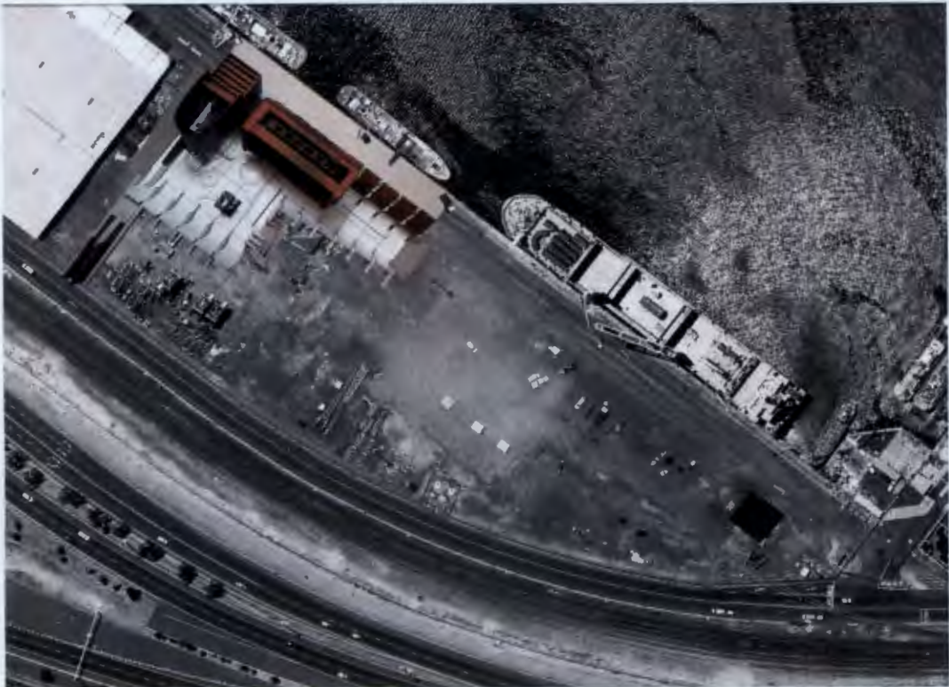
Fig. 07. Above: Isolated by highway and sea, KL-Berth is a concrete island. Fig. 08. Below: The project located within dock activity at KL-Berth.
