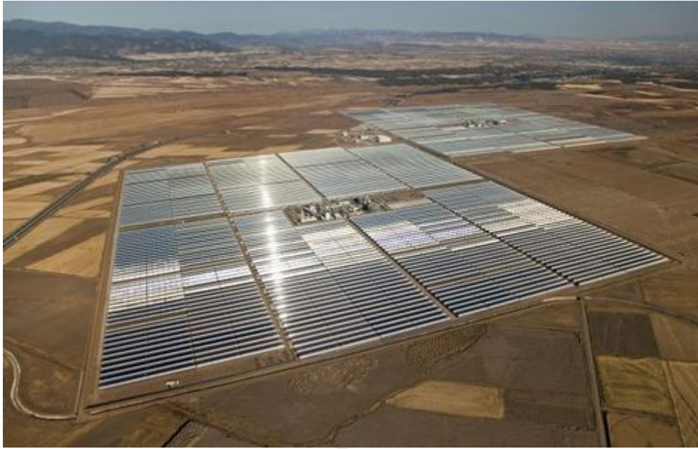
Figure 4-2 Andasol 1 parabolic trough technology plant
