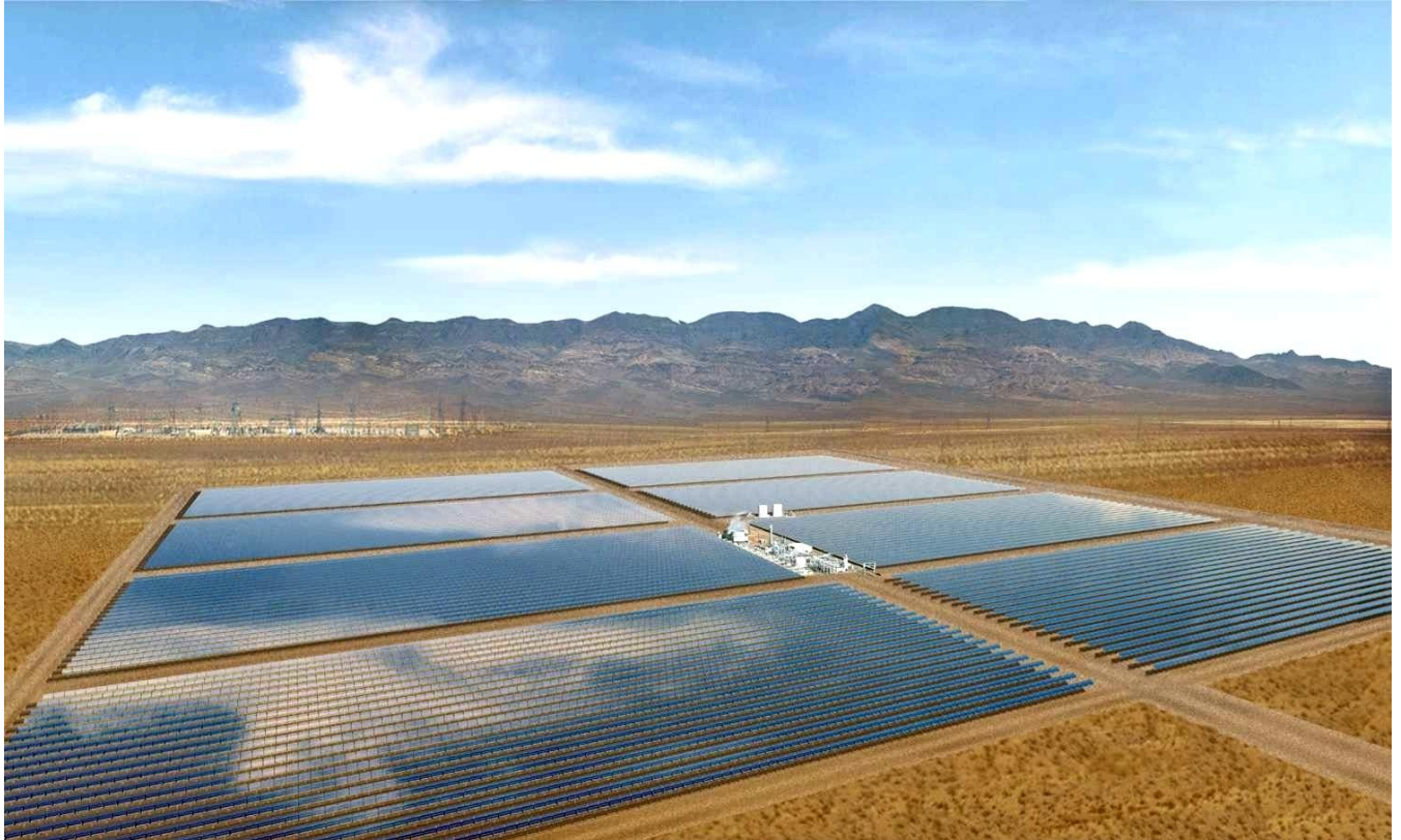
Figure 4-5 Aerial view of 64MW Nevada Solar One plant
