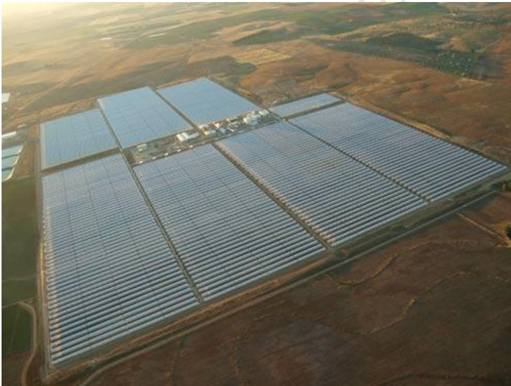
Figure 4-4 Aerial view of Alvarado 1 solar plant
