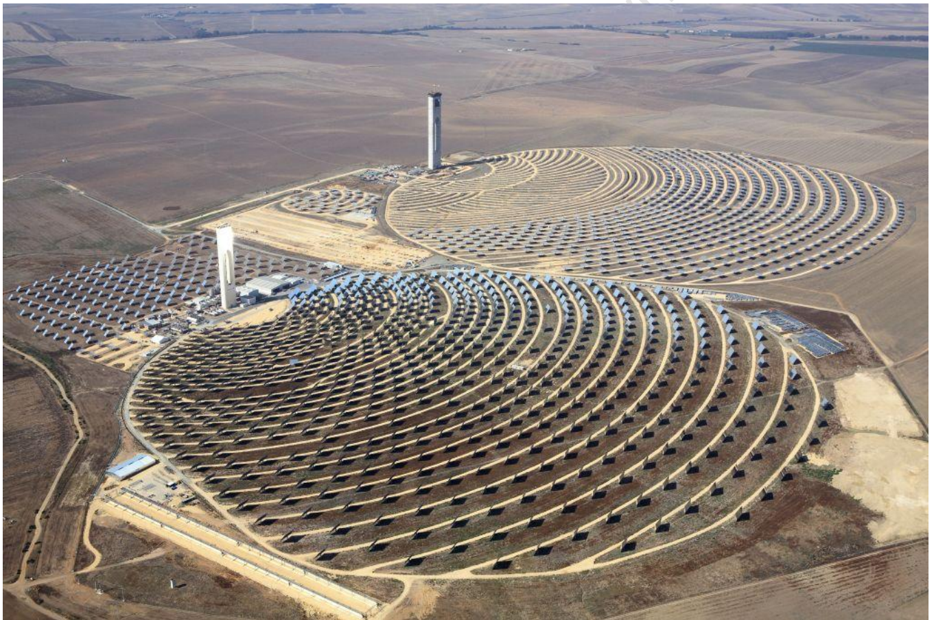
Figure 4-3 Aerial view of PS 10 and PS 20 solar tower technology plants
