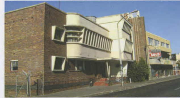
The Dutchess Factory, Victoria Road, Salt River
