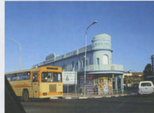
The bridge Mansions, Albert Road, Salt River
