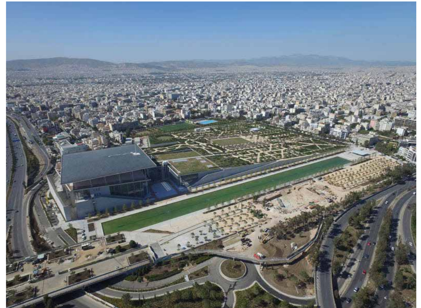
Figure 26: The SNFCC in its entirety (Renzo Piano Building Workshop, 2016.) Retrieved at: http://www.rpbw.com/all-projects
