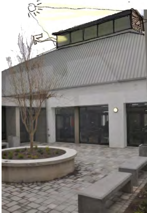
FIGURE 79. View from courtyard of roof monitor at Hermanus CDC. Image Credit: GLA.
