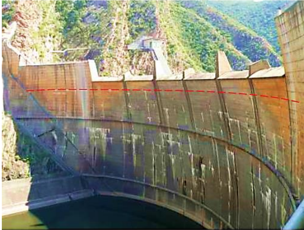
Figure 7.10: Approximate location of accelerometers within the gallery (adopted from Prins, 2017)
