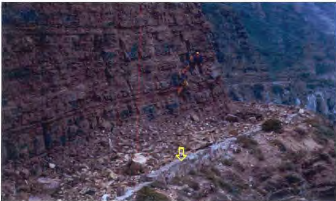
Plate 4.5: Barring activities released large amounts of slope material onto Chapman's Peak Drive making the identification of material falling after these activities had ceased very difficult. The arrow, indicating the road-side barrier, gives some indication to the depth of material left on the surface of the Drive (5/3/2000).
