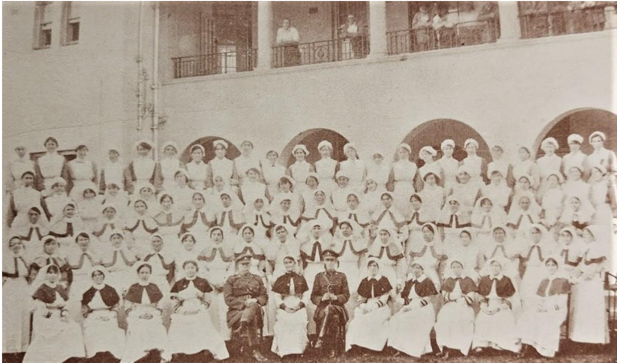
Photograph 33: Nursing staff, Alexandra Hospital, Maitland
