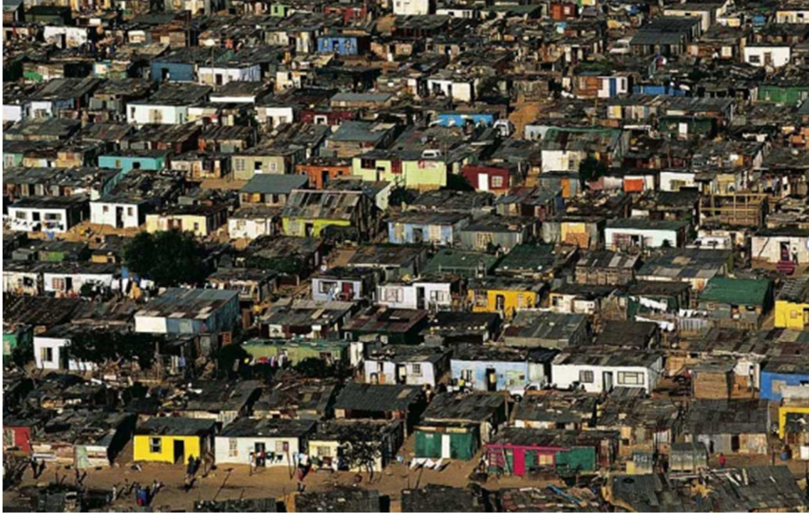
Figure 3.3: A part of Soweto with government funded houses and the informal houses known as shacks
