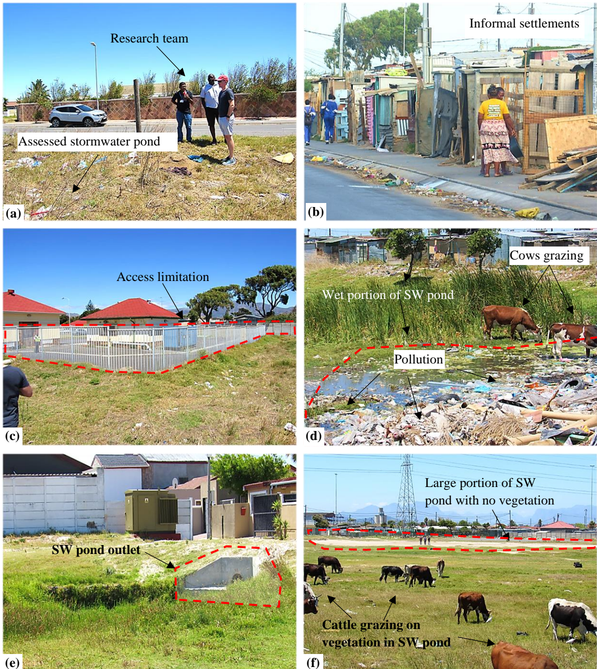
Figure 4-1: Images of study area captured during preliminary site investigation of SW ponds
