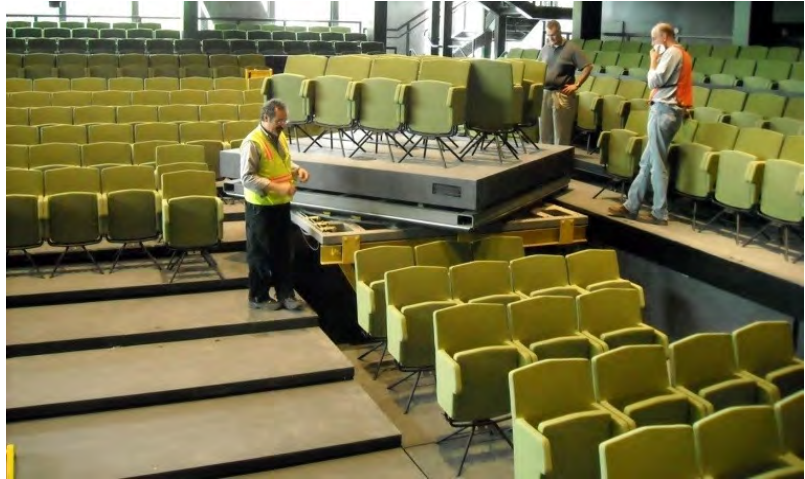
Figure 10 A floor element being moved into position through rotation.
