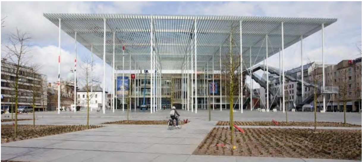
Figure 34 Theatre Square's steel frame structure touching the ground 'lightly'.
