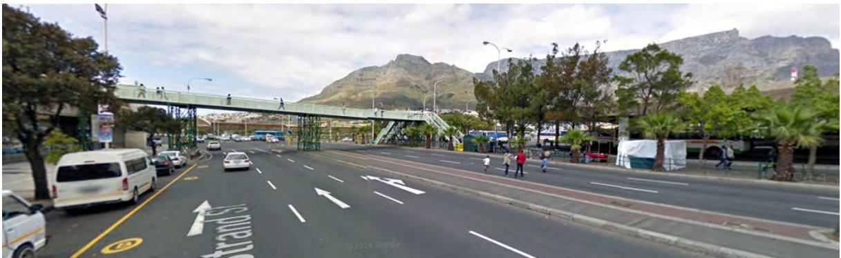
Figure 25 Station deck's pedestrian bridge crossing Strand Street before dropping pedestrians off before the Golden Arrow bus depot.
