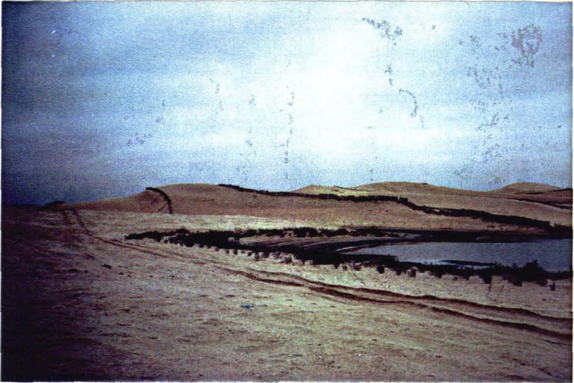
Plate 20 Dune stabilisation south of Walvis Bay Town undertaken by the Directorate of Forestry - pole-barriers, vegetation plantings and flooding of interdune areas.
