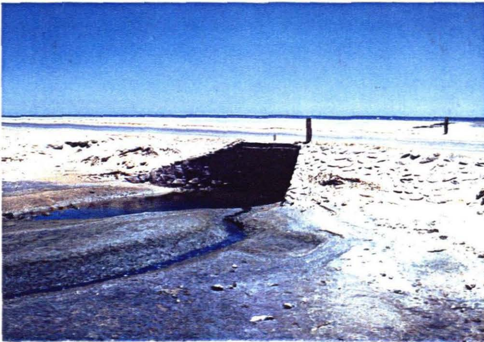
Plate 21 A sluice that controls the movement of water into dune areas, with the Walvis Bay Lagoon in background.
