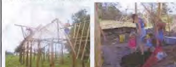
Fig 77 KnulaDhamma timber frame and members making earth mixture
