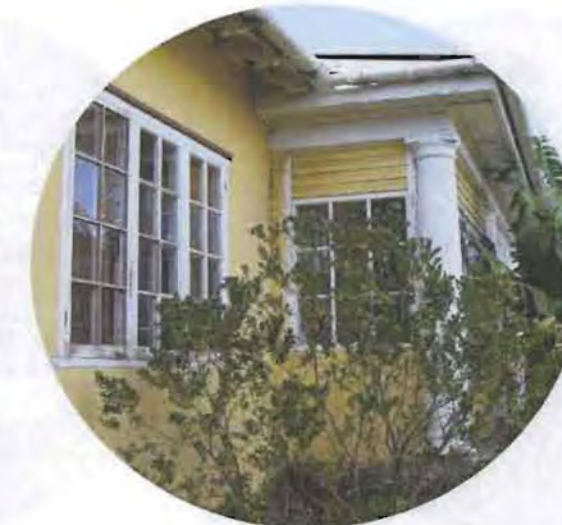
Resident house Q1(former doctors house)
