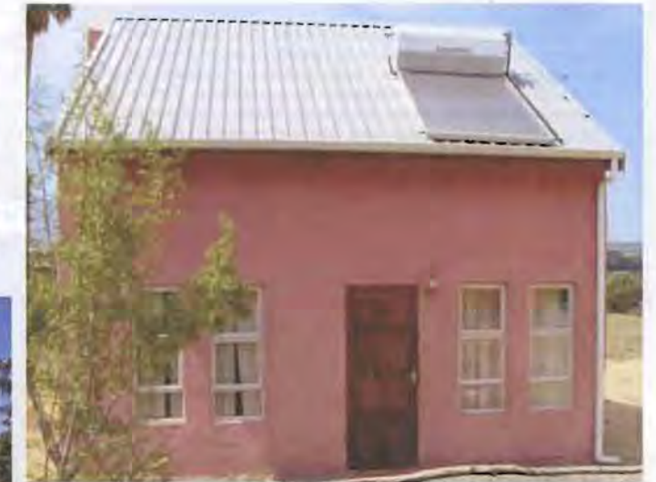
Fig 48 Lynedoch, house with solar power panel
