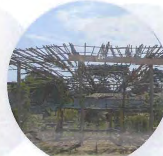
Shade structure next to Youth Garden
