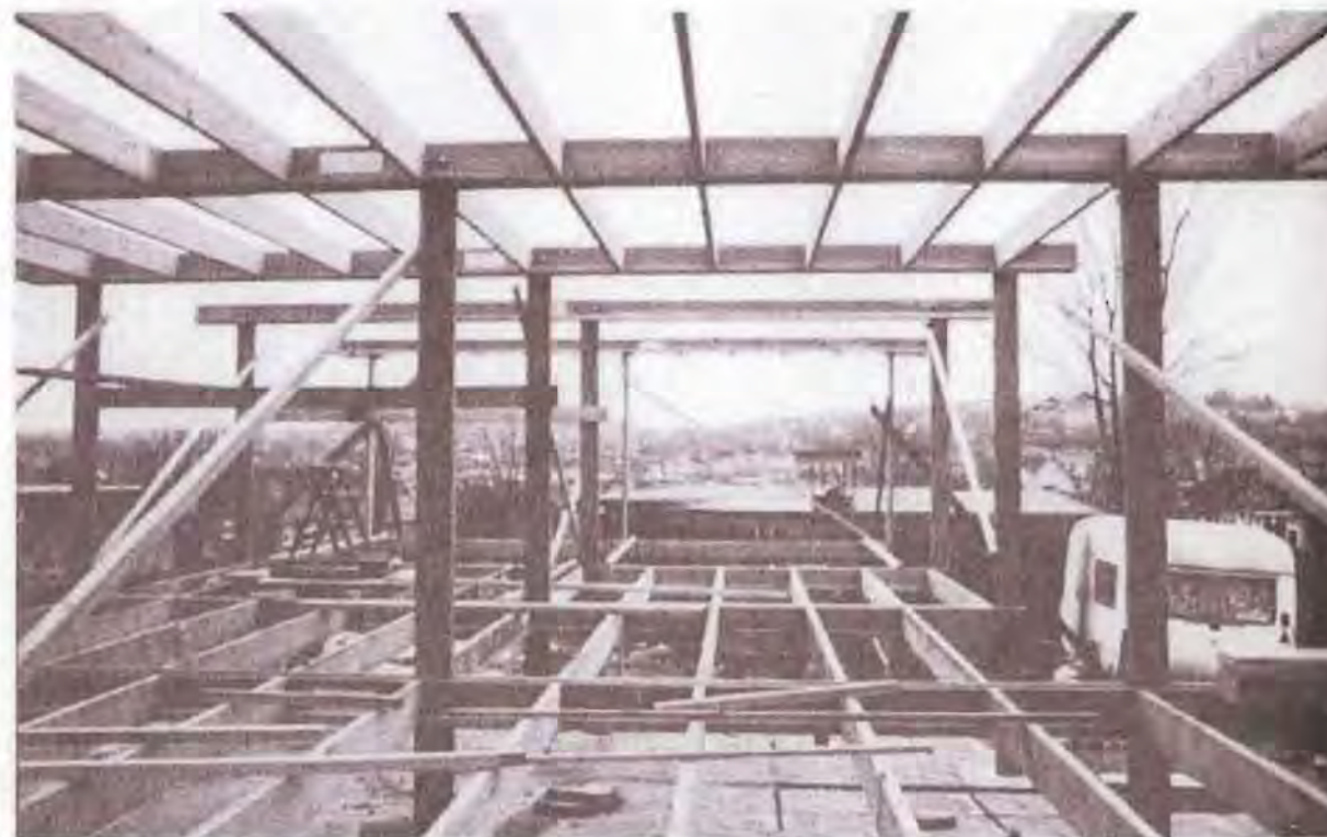
Fig 33, 34,35 Timber framed structure
