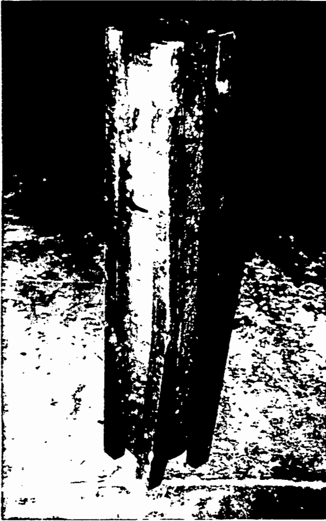
Fig. 7.9a: Timber Frame with Concrete Cylinders - Tidal Zone
