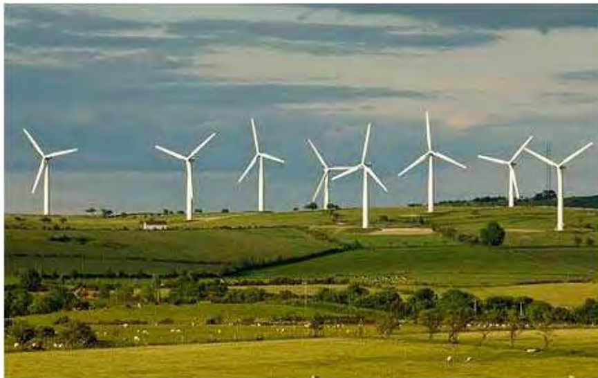
Figure 2-3. Example of a large wind farm [59]
