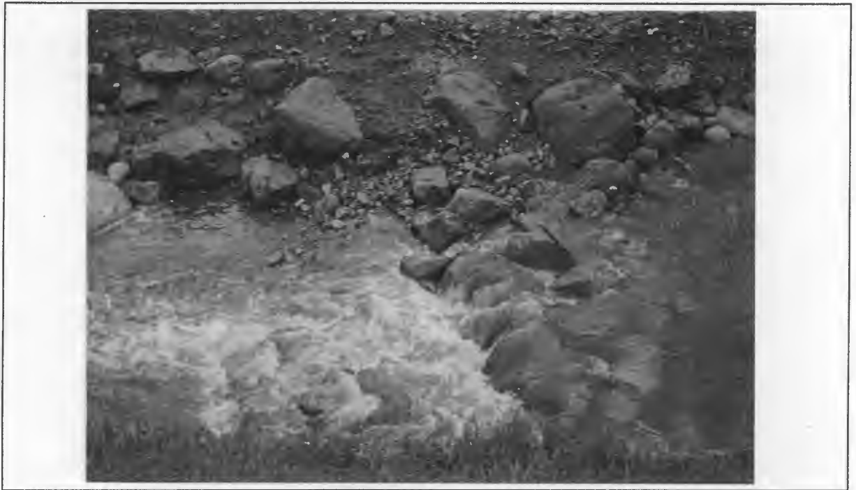
Figure 8.8: A number of boulder weirs should be constructed in the upper Liesbeek River to control bed degradation
