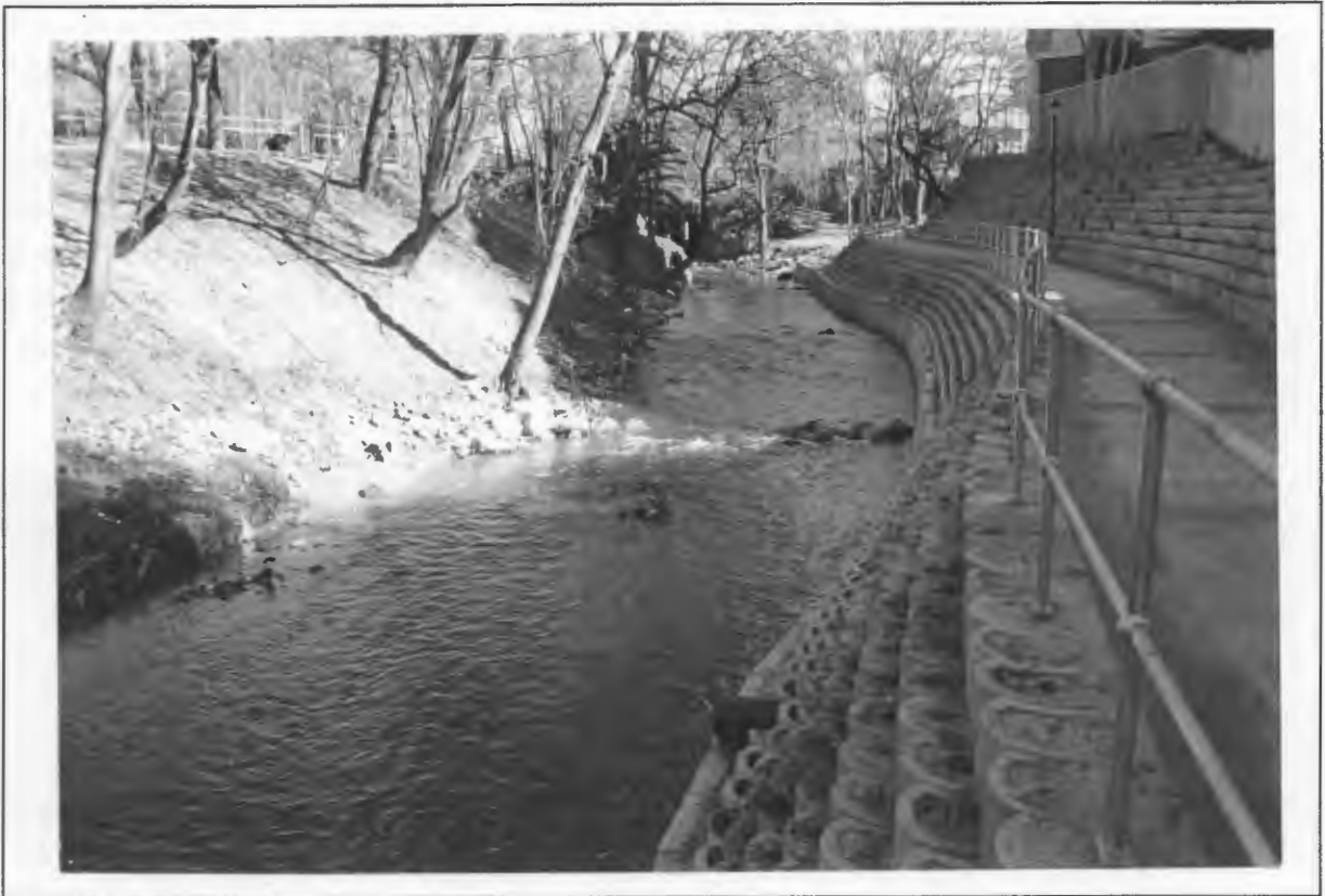
Figure 8.5: The Southern Life section of the Liesbeek River walkway has increased the amenity value of the corridor
