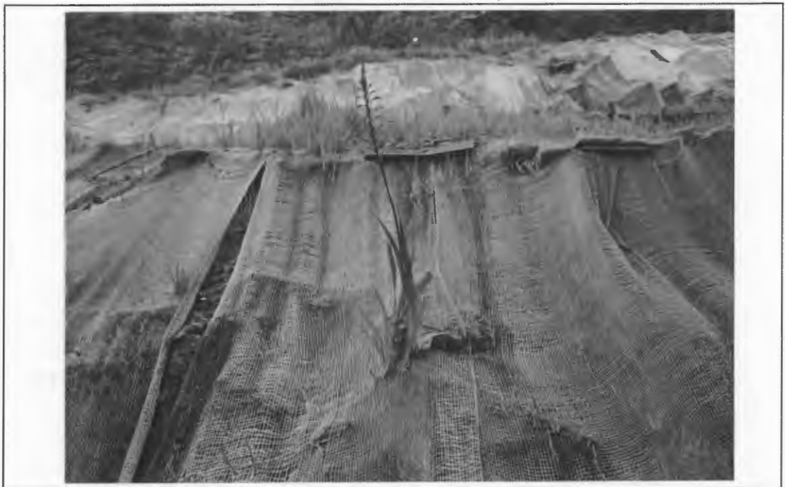
Figure 7.11: Biodegradable geotextile mesh assists the establishment of vegetation and allows the plants to grow through
