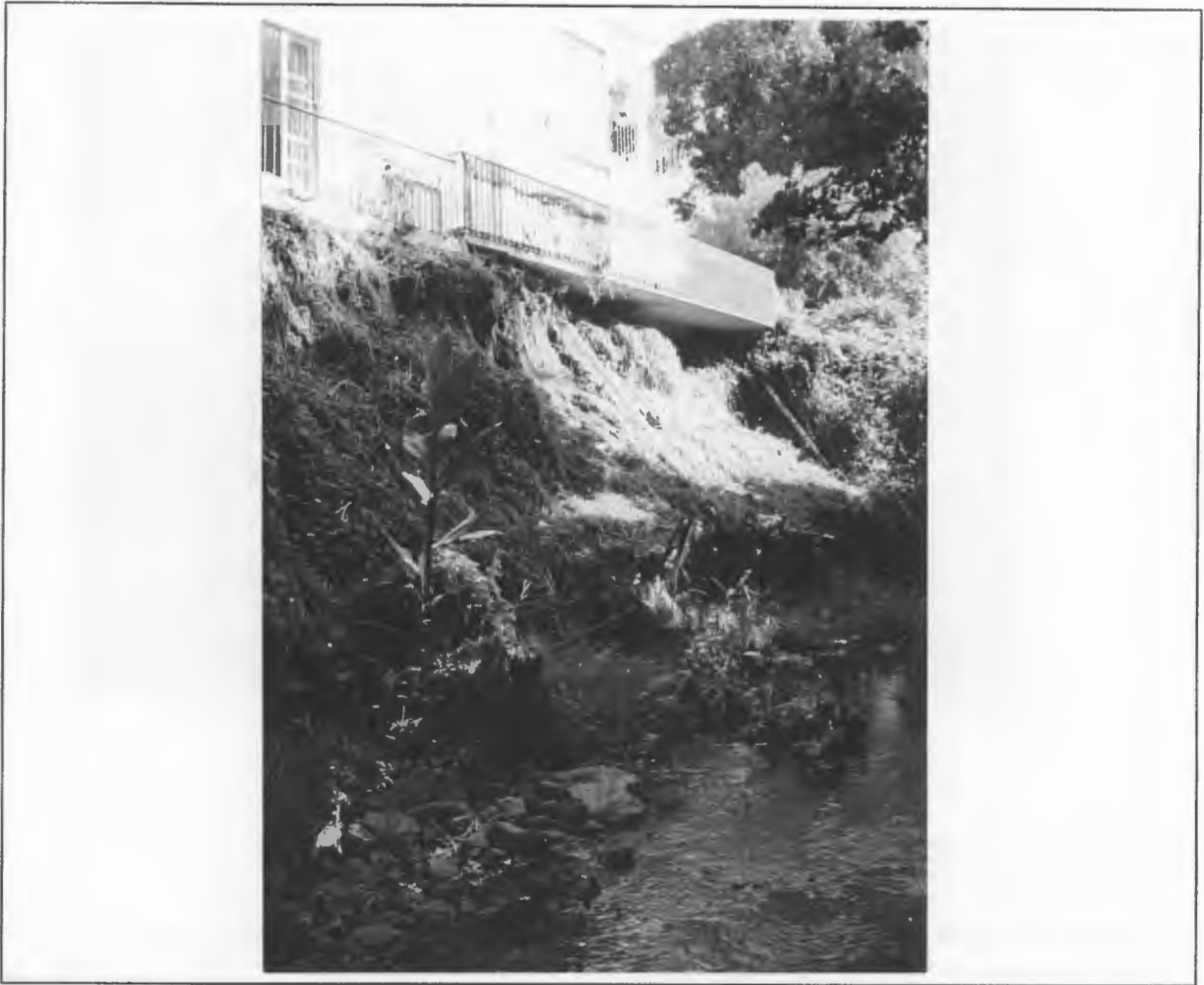
Figure 8.6: Urban development close to the river channel forecloses environmentally-sensitive options and requires that the banks are stabilised
