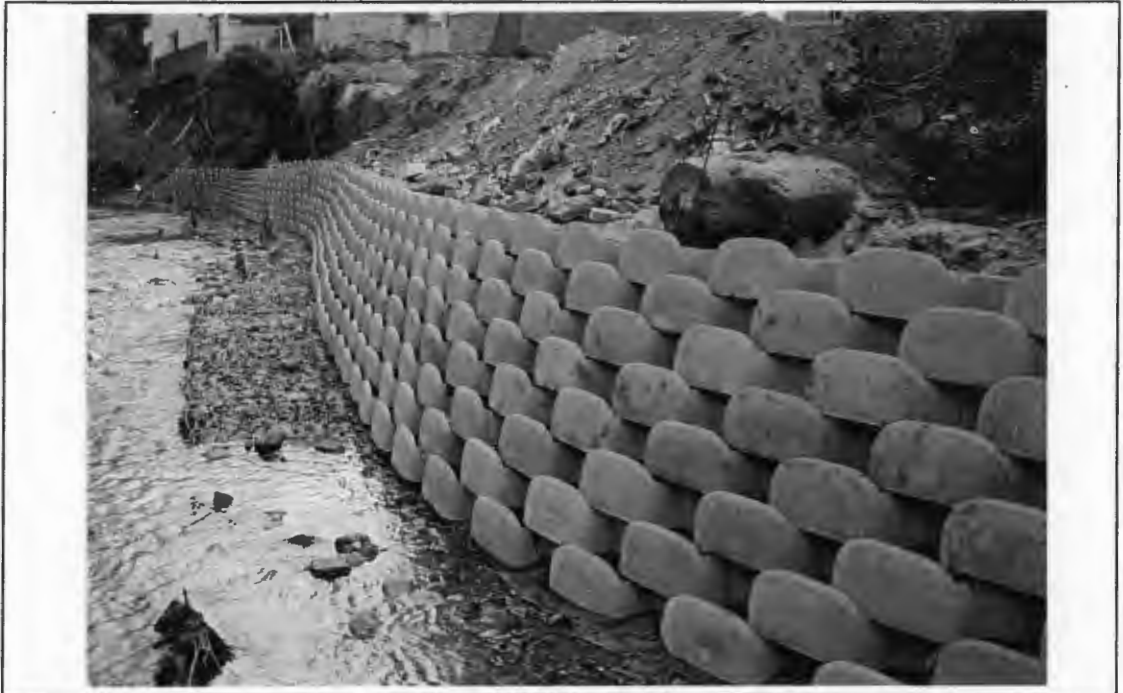
Figure 7.8: There are numerous types of cellular concrete revetments available: the "Waterloffel" shown here has limited soil space and no drainage holes
