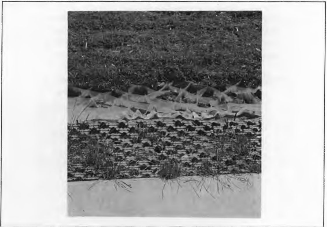
Figure 7.9: Preformed "Hyson" cells can be filled with concrete, or with topsoil prior to seeding the banks with grass
