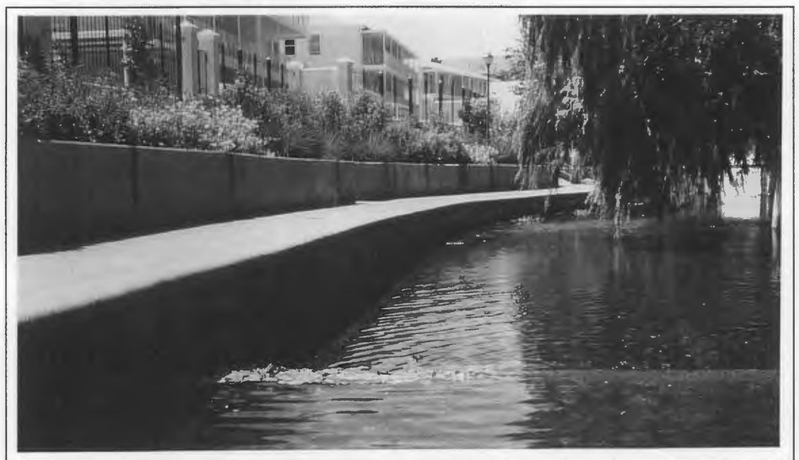
Figure 7.29: Channels which do not convey flows on a regular basis can be used for amenity purposes
