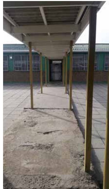
4 Covered walkway across school
