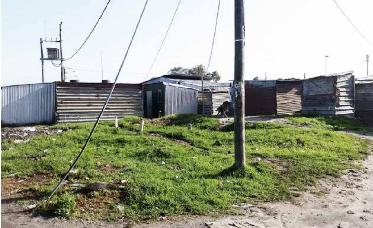
2 Type of water point inside informal pocket open space in Barcelona
