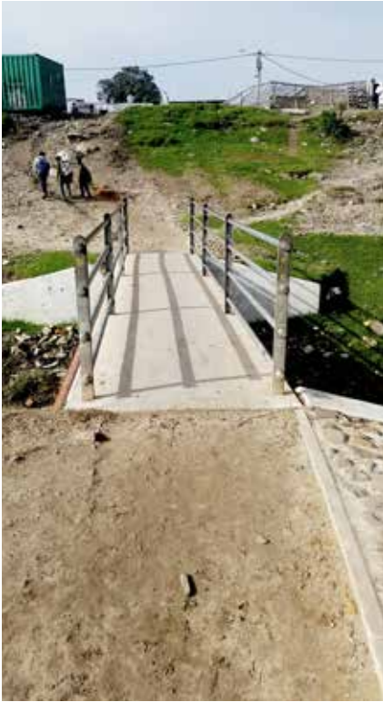
2 Bridge over canal
