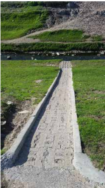
2 Access over canal
