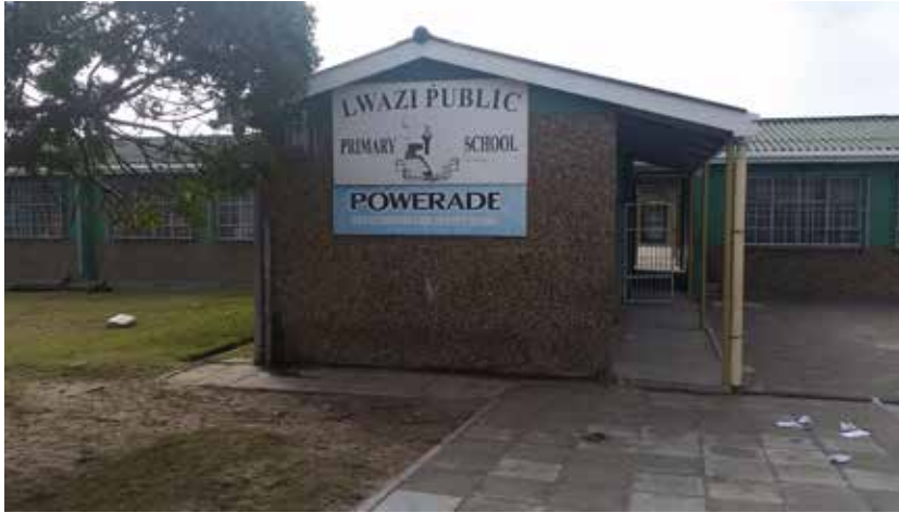
1 Entrance from Klipfontein Rd
