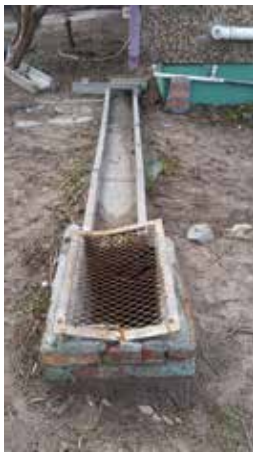
3 Rainwater drainage condition
