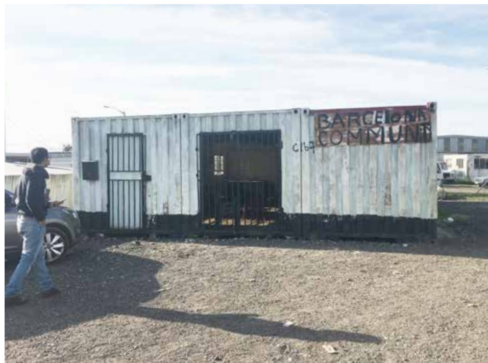
2 Entrance of hall accessed through metal burglar door with no enclosure
