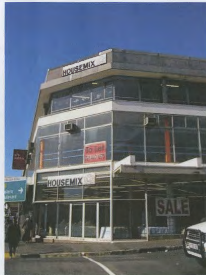
BELOW: The orientation of shop fronts along Main Road aid in their economic sustainability.
