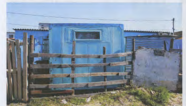
Metal sheets from industrial fridges are used as cladding
