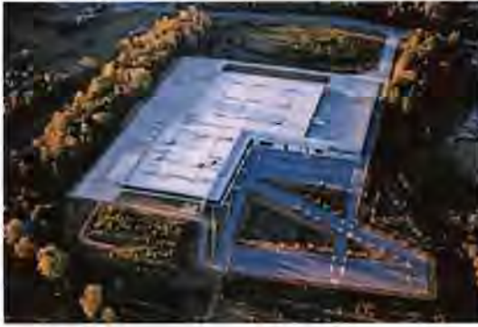
Top left: The constructed wetland of the Herman Miller Factory, with a ground plane articulated by soft and hard surfaces
