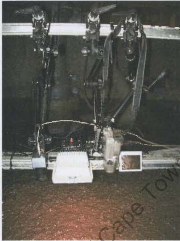
Figure 3.45: SmartFroth camera and lighting system installed on rougher 3 of the molybdenum circuit.
