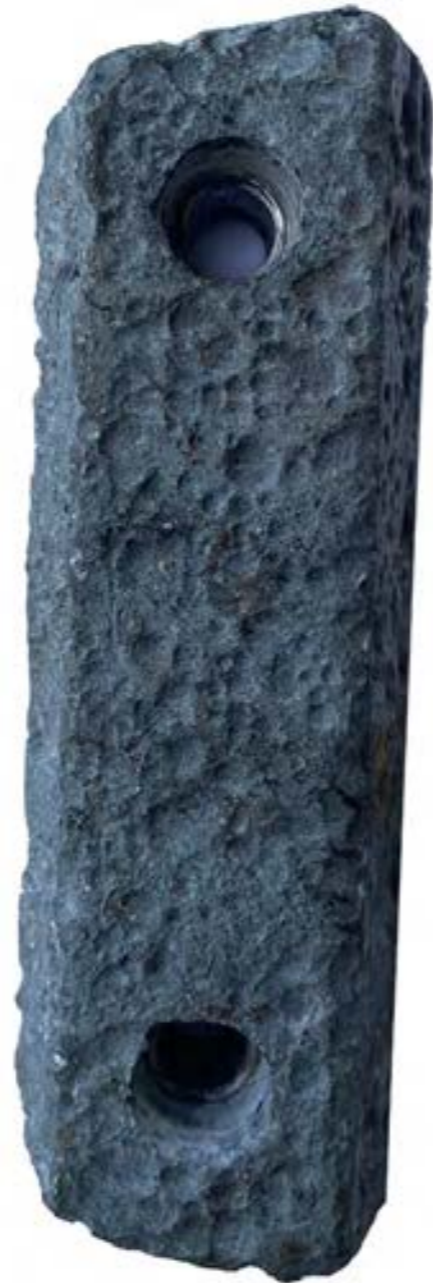
Fig. 20. Documenting weathered concrete found near the harbor
