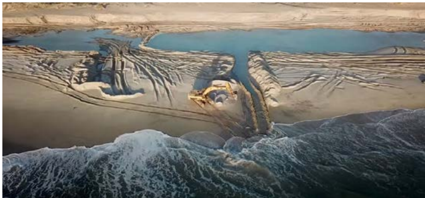
Fig. 28. Excavating beach sand
