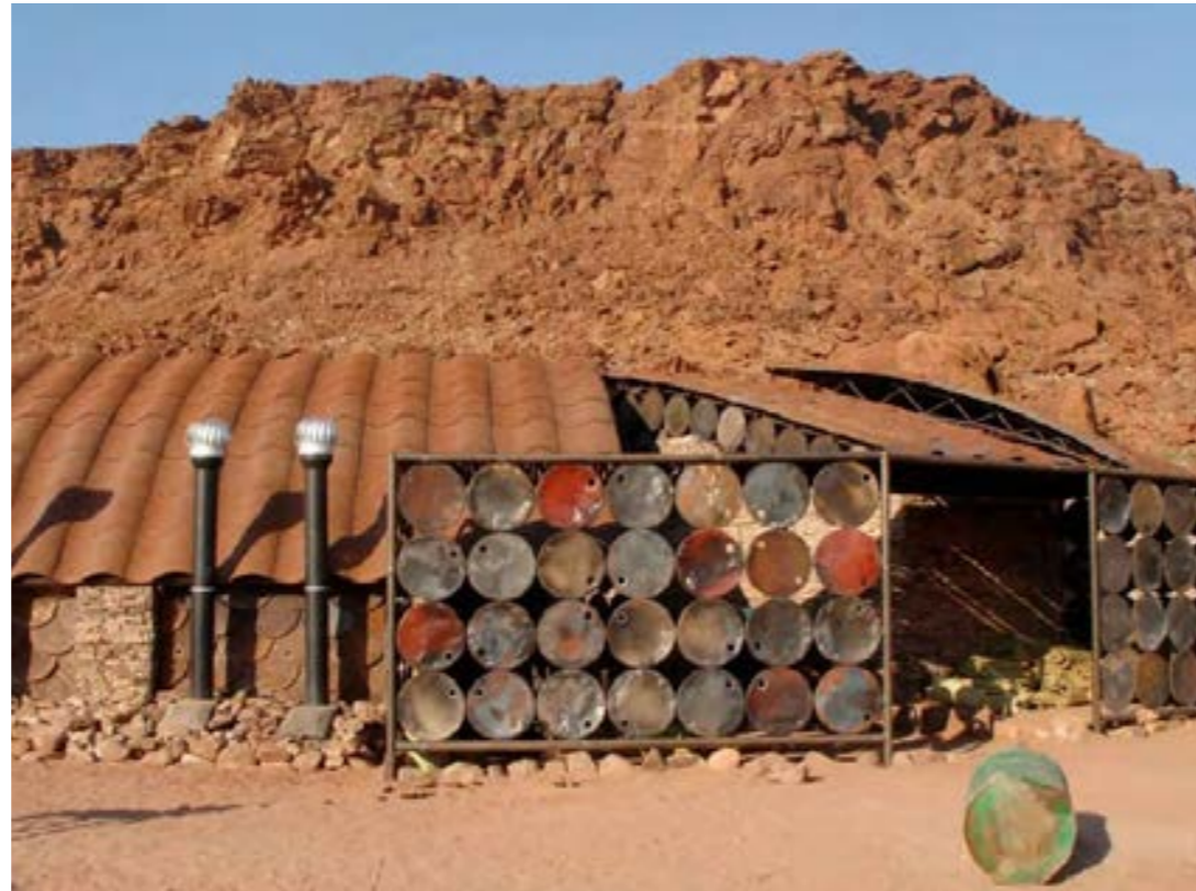
Fig. 17. Decayed oil drums regenerated to a facade Nina Maritz. Twyfelfontein Visitor's centre (2005 - 2007).
