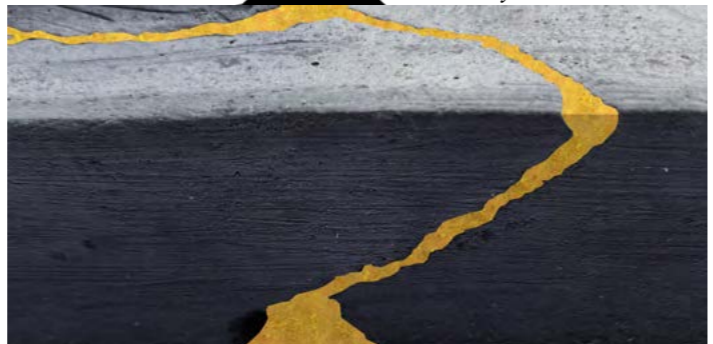
Fig. 15. Restoring the crack of model A
