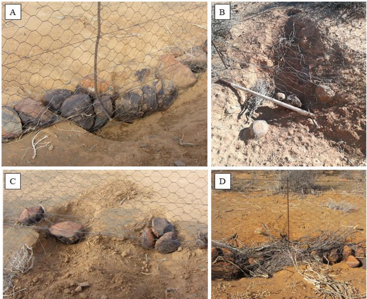
Figure 6.3: Example of holes repaired with rocks (A and C), or branches and poles (B and C).
