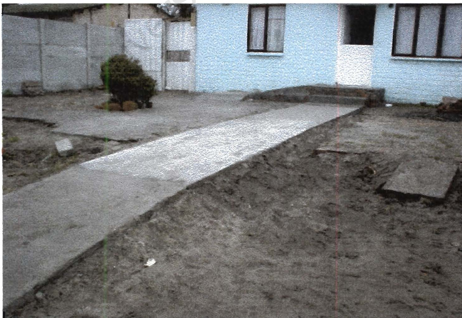
Photograph 7: Concrete ramp from front door and pathway leading to road
