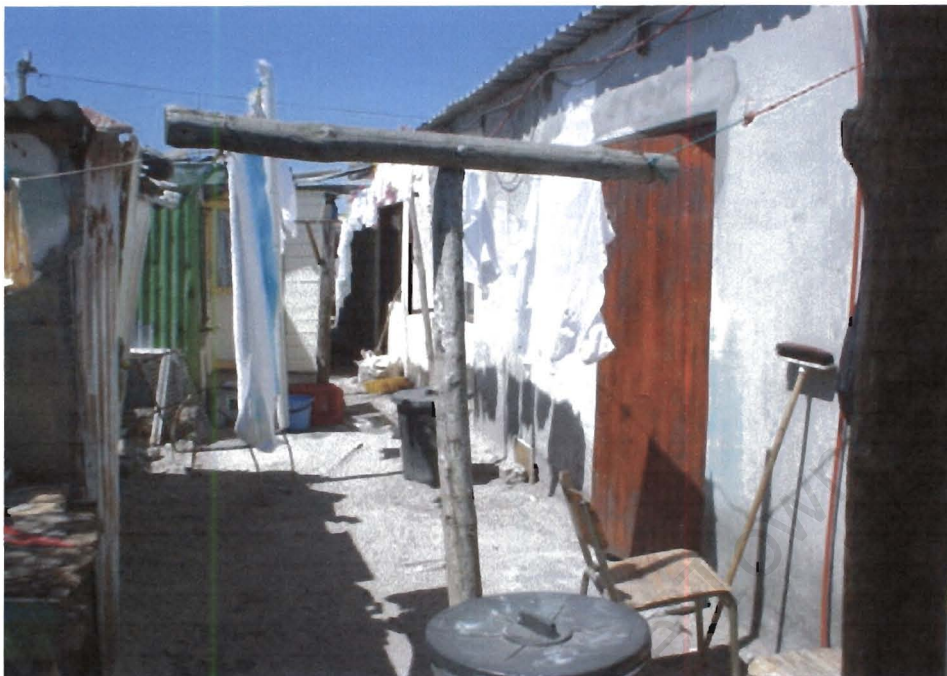
Photograph 11: Backyard shacks of semi-detached house accommodating four families
