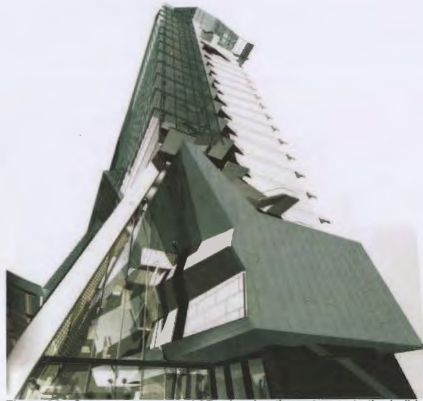
Figure 38_ Computer generated 3D, showing the entrance to the building. The layering of the facade can be seen from this image, and how the scrim skin wraps itself over the building.
