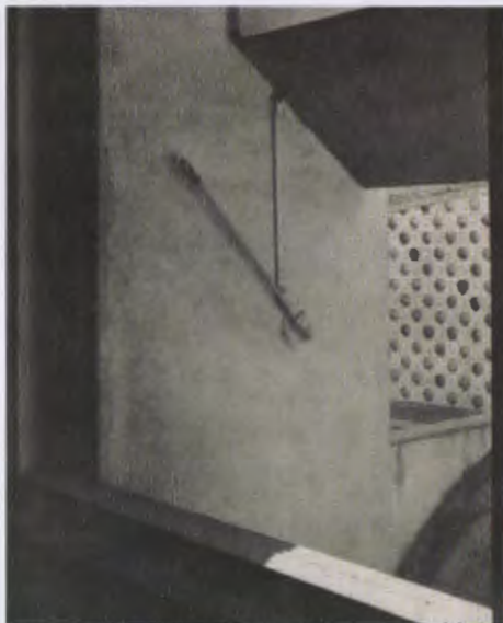
Figure 36_ Interior photograph looking out onto the sunshade and adjustable horizontal asbestos louvres
