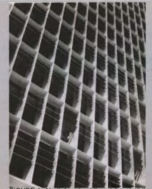
FIGURE 4 _North facade of the ministry building
