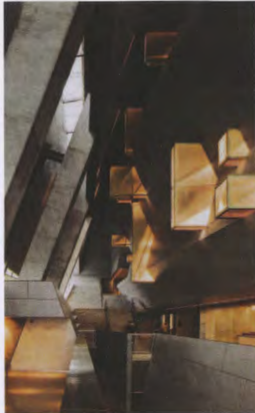
FIGURE 7 _ interior view of entrance to San Francisco Federal building
