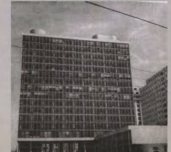
FIGURE 5 _South facade of the ministry building
