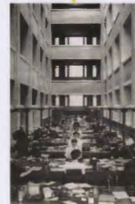
Larkin building, Frank Lloyd-Wright
