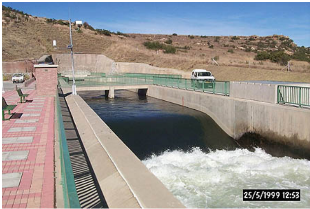
(a) Katse outlet tunnel 4
