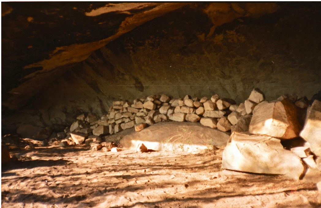
Figure 8.3: A view of the stone walling on top of the roof fall.
