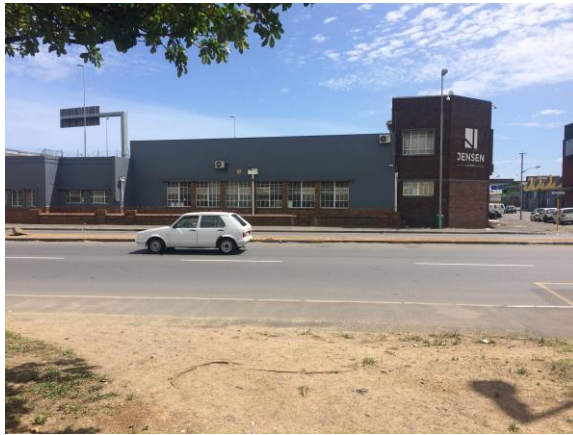
[9] Lack of street frontage at the industrial Jensen Belts building
