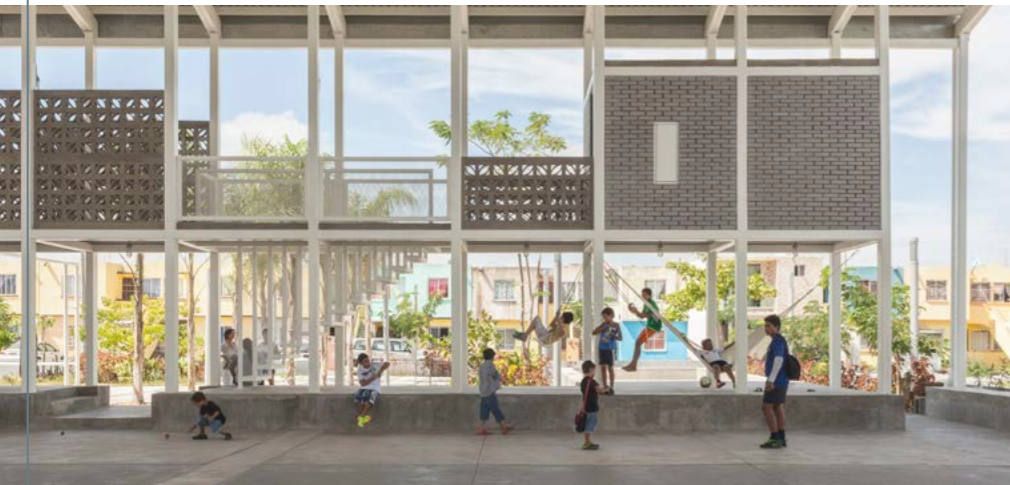
Figure 158: This Community Center in Boca del Río, Mexico, was once an open and disused asphalt lot, located on the periphery of a marginalised settlement. The structure provided shade from the elements, and created a space where an assemblage of uses could take place.
