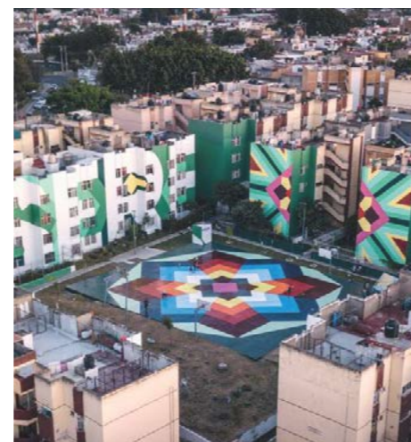
Figure 167, and Figure 168: (Below) The project "was conceived collaboratively... the work and it's development like a transgenerational mirror. A place built on bridges between different social realities working together. This way of building cities should be a model today, in order to develop the society of the future" (Guerra, et al., 2018, 22). This treatment of public housing illustrates the potential in upgrading, with limited budget, the dignity of spaces and housing.
