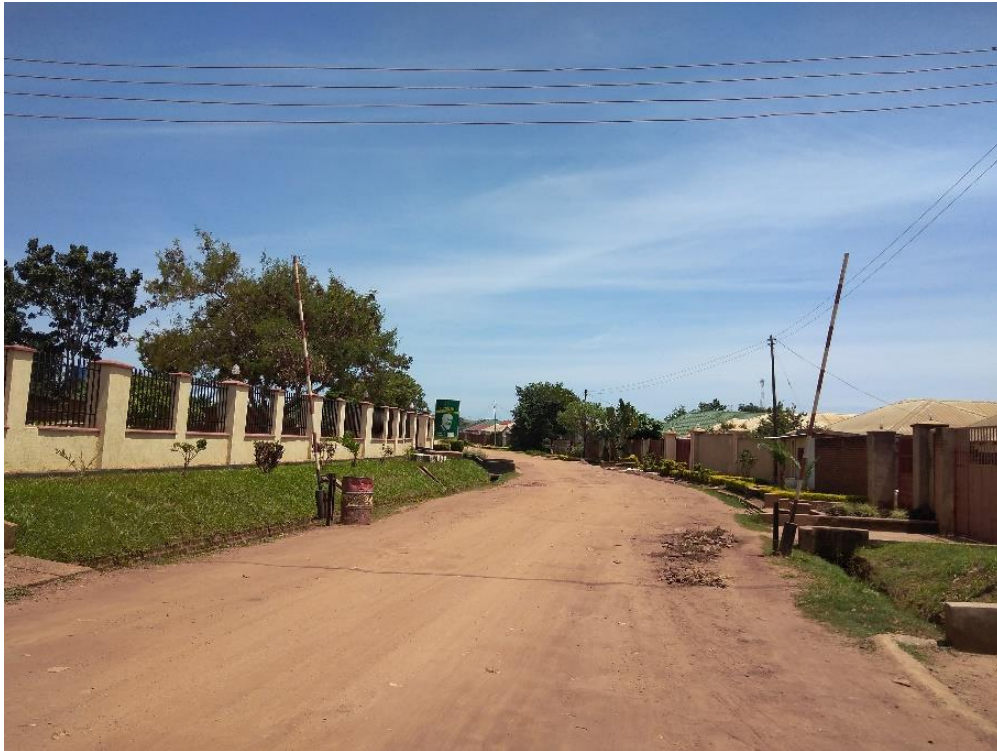
Figure 1: A section of Gulliver Street, Area 49
