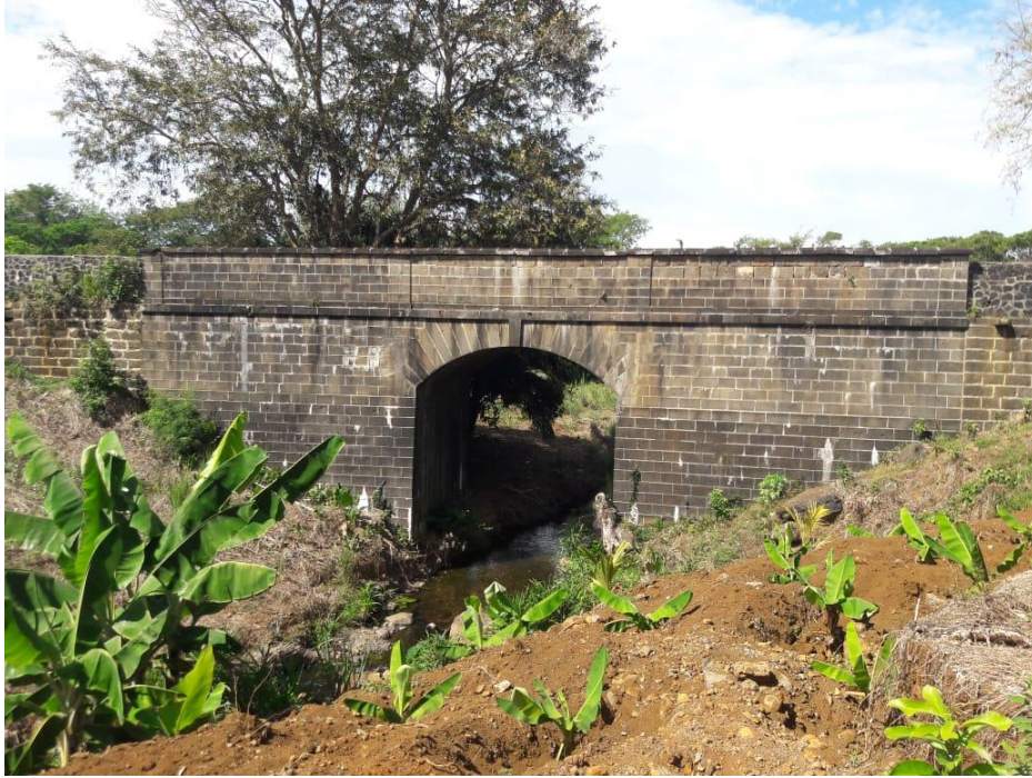
Figure 4: Courtesy of Moshumee T. Dewoo. 'Bain des Nègresses' railway-bridge.
