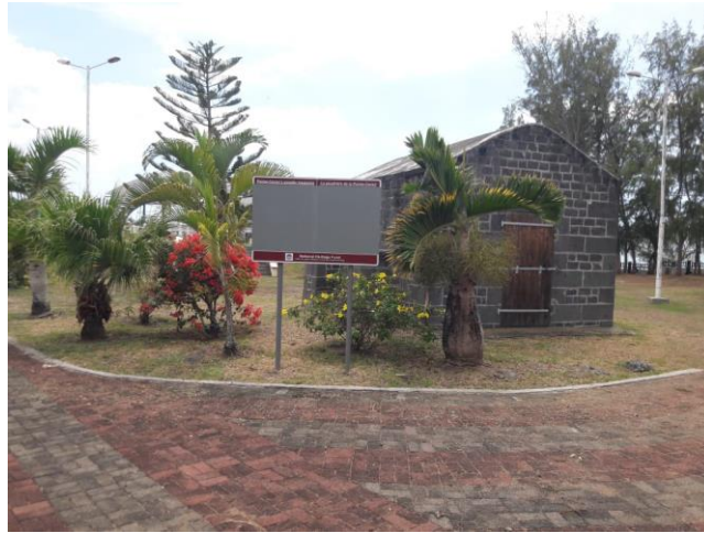
Figure 9: Photo Courtesy of Moshumee. T. Dewoo. National Heritage Building.
