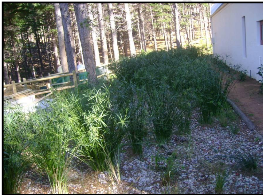
Figure 7: Constructed wetland at De Goede Hoop Estate (western view)
