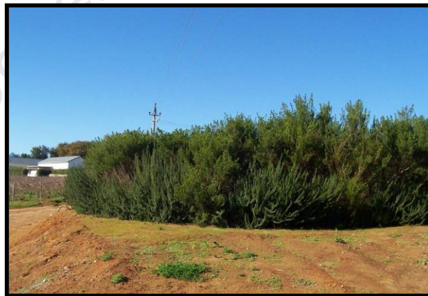
Figure 9: Constructed wetland at Wolwedans Farm (southern view)
