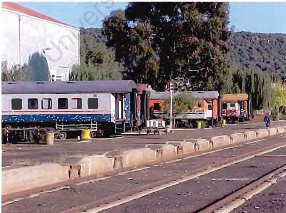
THE TRANSWERK COACH REFURBISHING PLANT AT BLOEMFONTEIN
