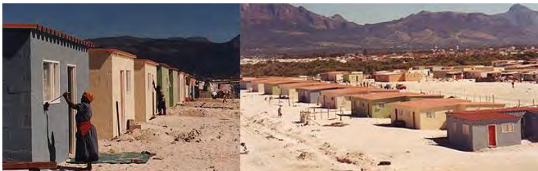
Figure 5: Photographs of formal houses being completed in March 2000 (Source: Schrire, n.d.).
