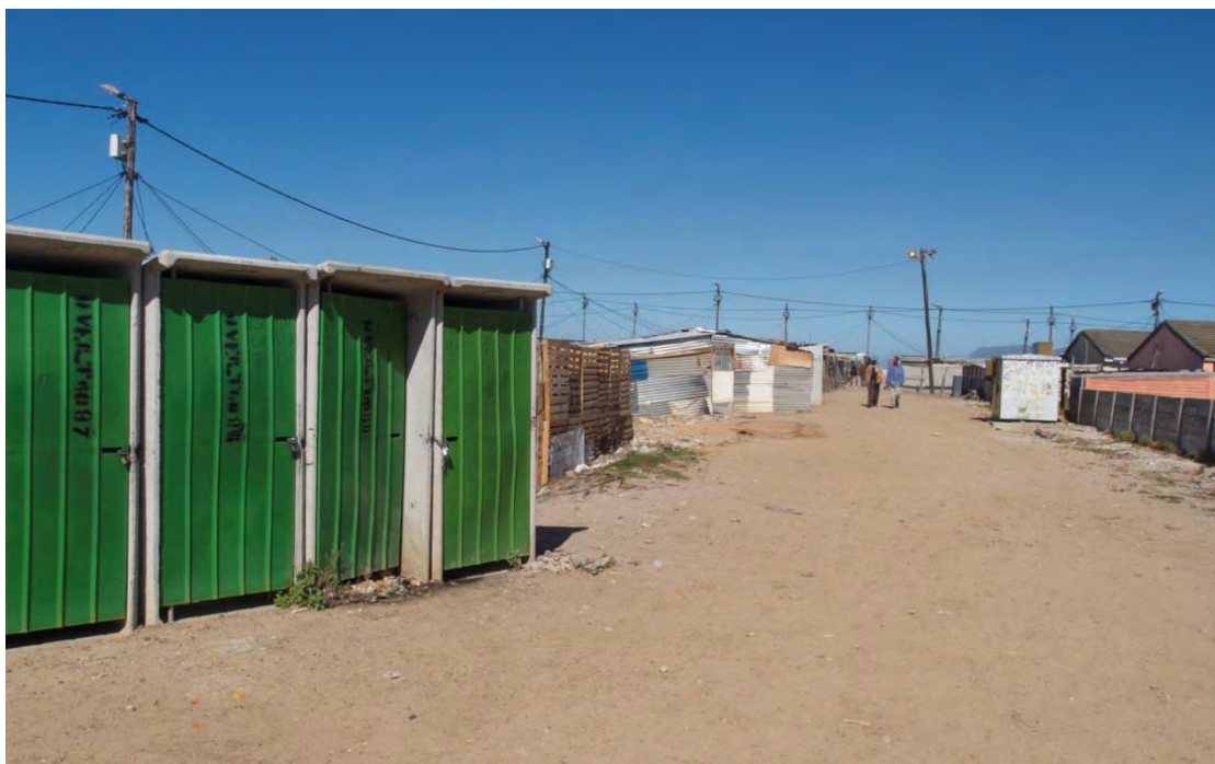
Figure 19: Communal flush toilets located on an informal road in Overcome Heights
