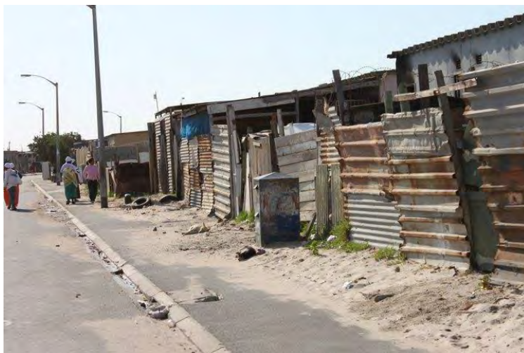
Figure 3: Vrygrond streetscape (Davies, 2013)
