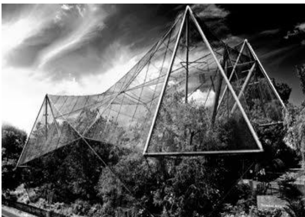
Fig34: Photograph tensile structure
