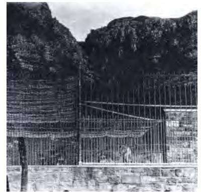
Fig 18: Caged barrier condition
